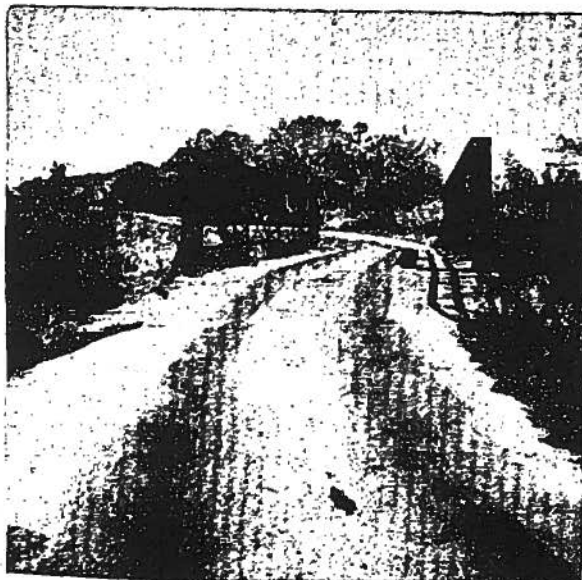
Figure 2. Note missing bridge railing at left.
