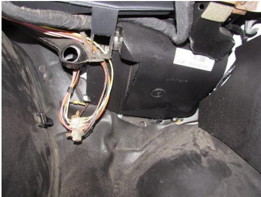
View of HVAC from interior
