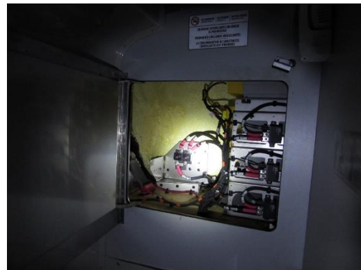
Cavity behind the lavatory mirror
