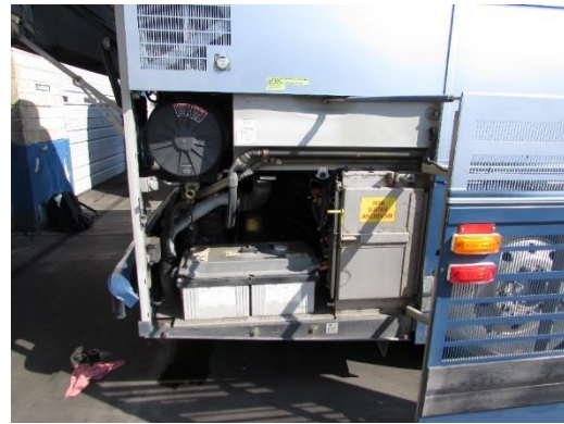
Side view showing toilet tank
