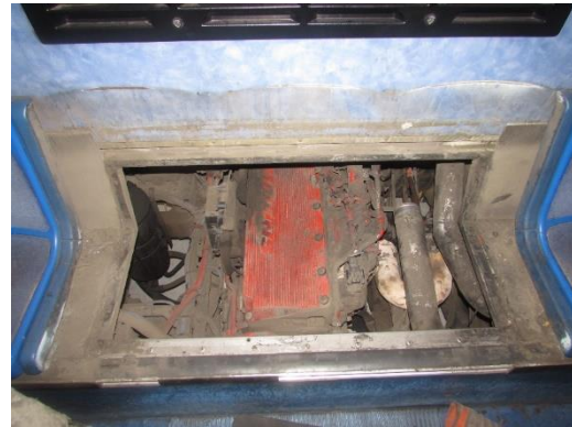
Engine access panel
