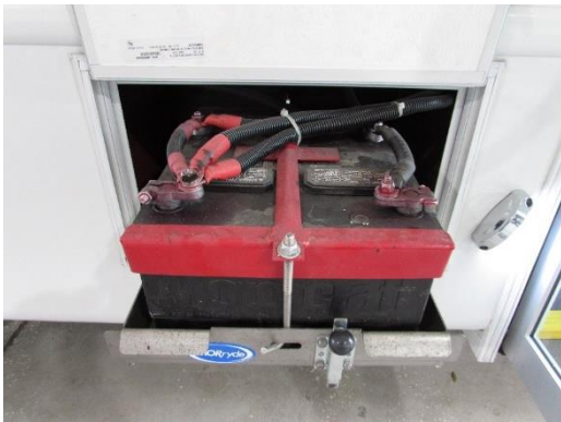
View of battery compartment on passenger side of vehicle
