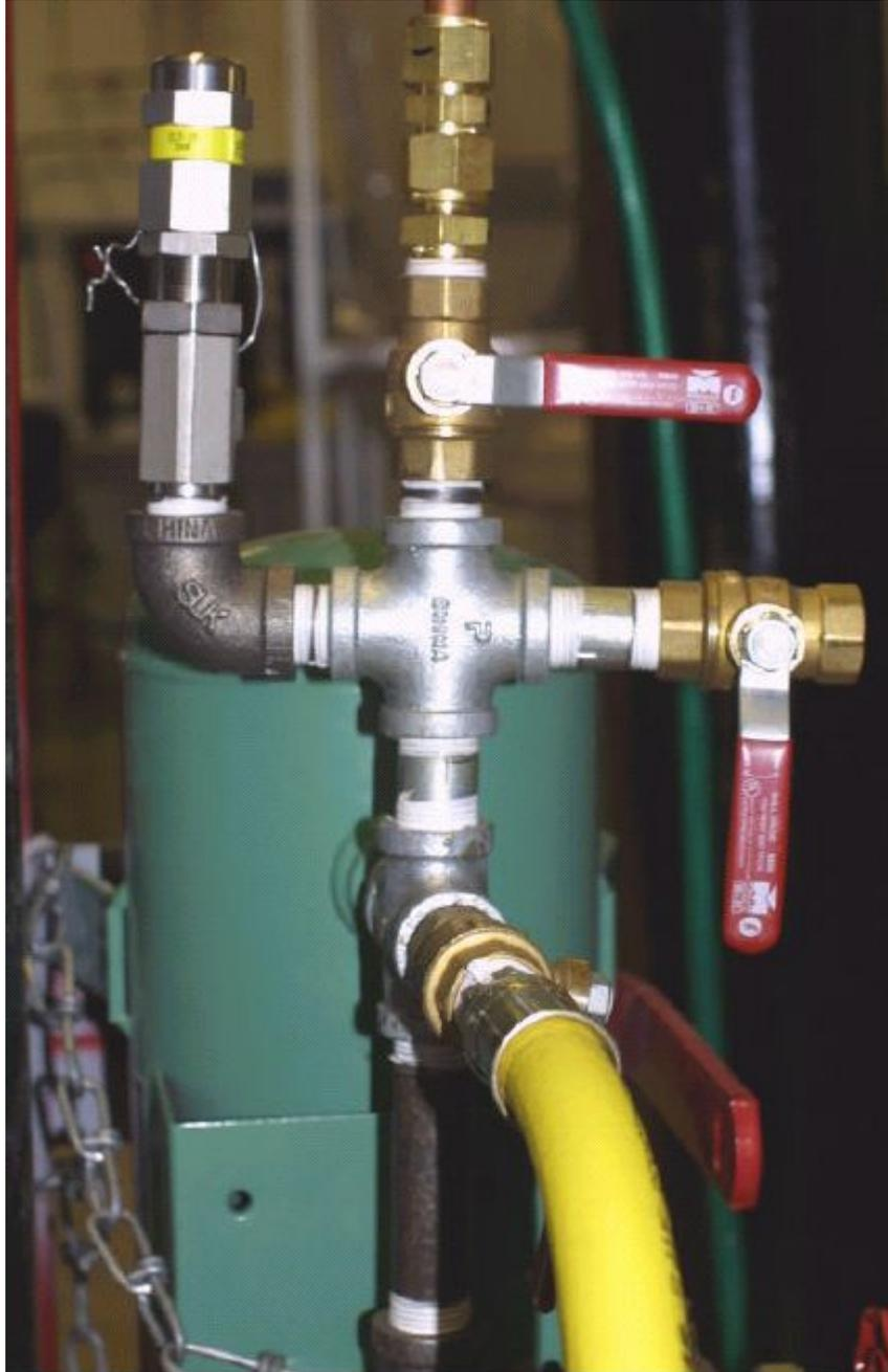
Figure 5: Cross-Junctions on Nitrogen Flow Lines
